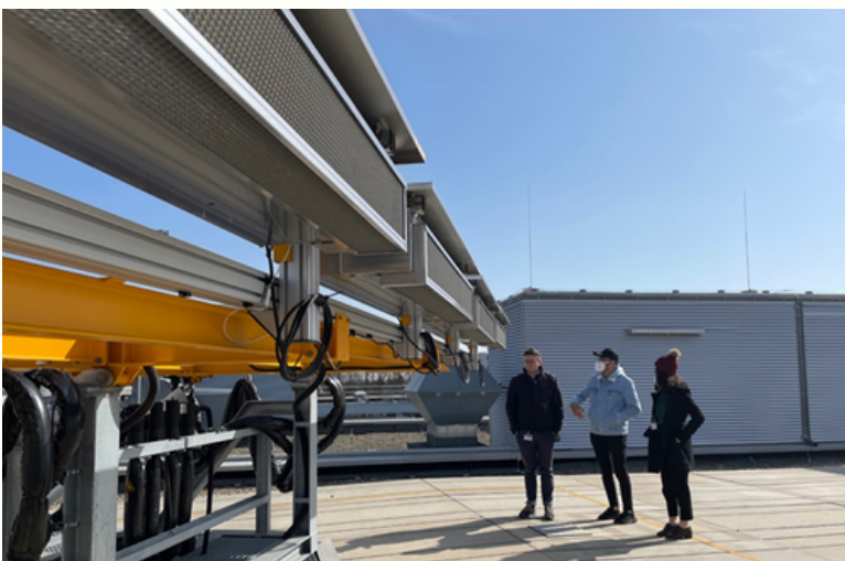
Mrs D. Nouicer, Mr Fedi Abdellaoui and Dr M. Ehrenwirth on the rooftop of THI, where, among other things, a solar thermal tracker (right) and steel structures (right) for flexible PV and solar thermal modules are installed.
